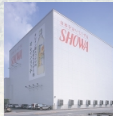
Funabashi Distribution Center
